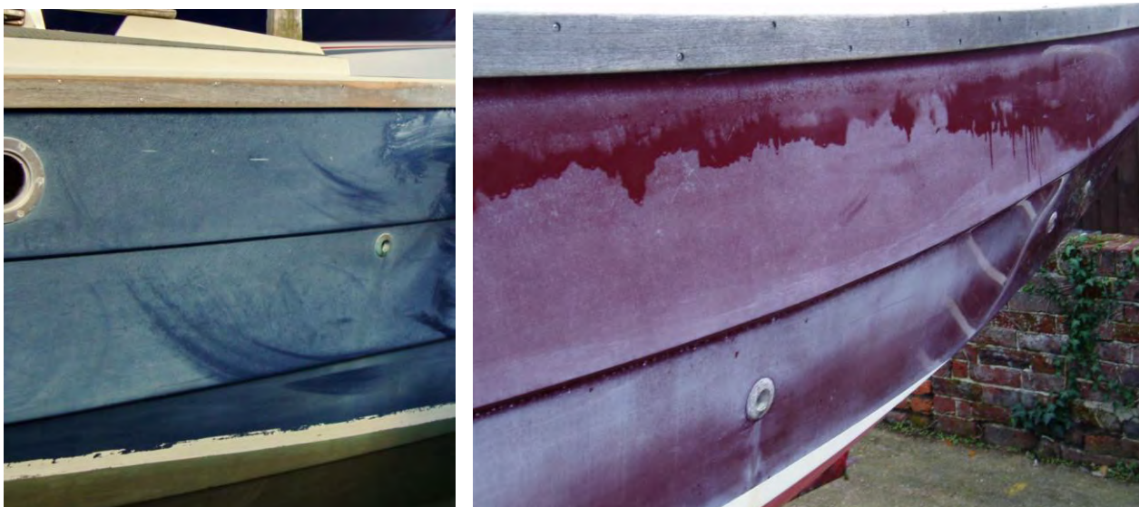
Hulls requiring Deep Cut
